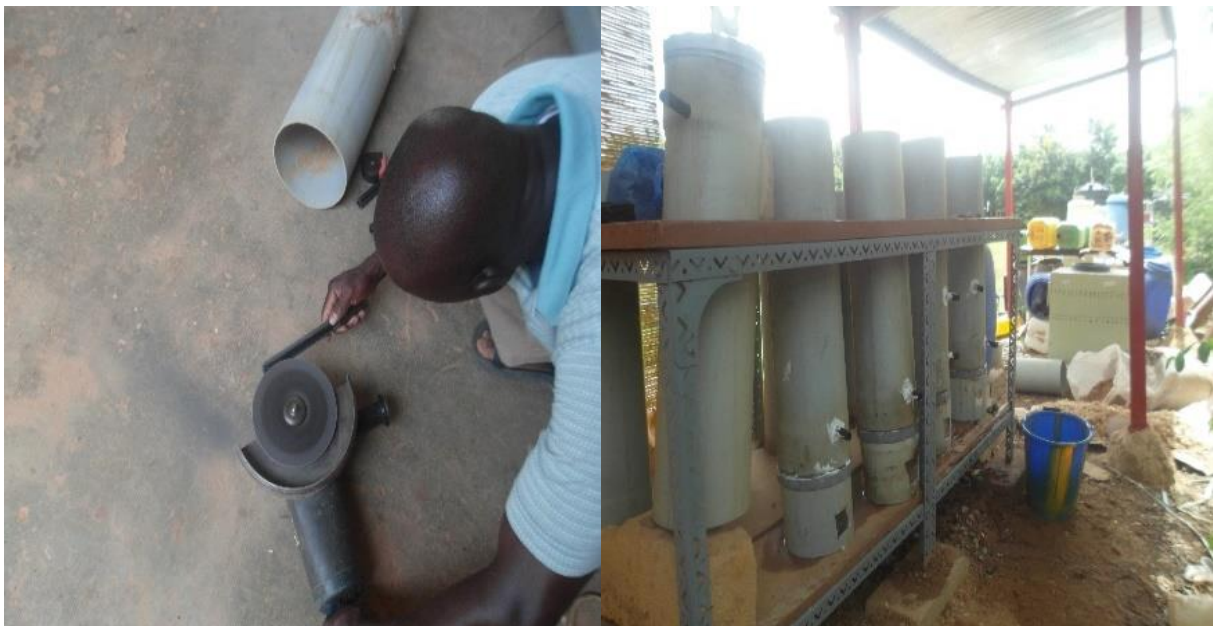
(a) Construction of filters
