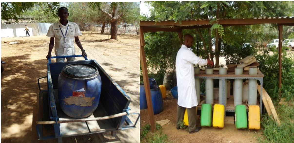
Figure 3-4. Greywater collection and supply to the vermifiltration system
