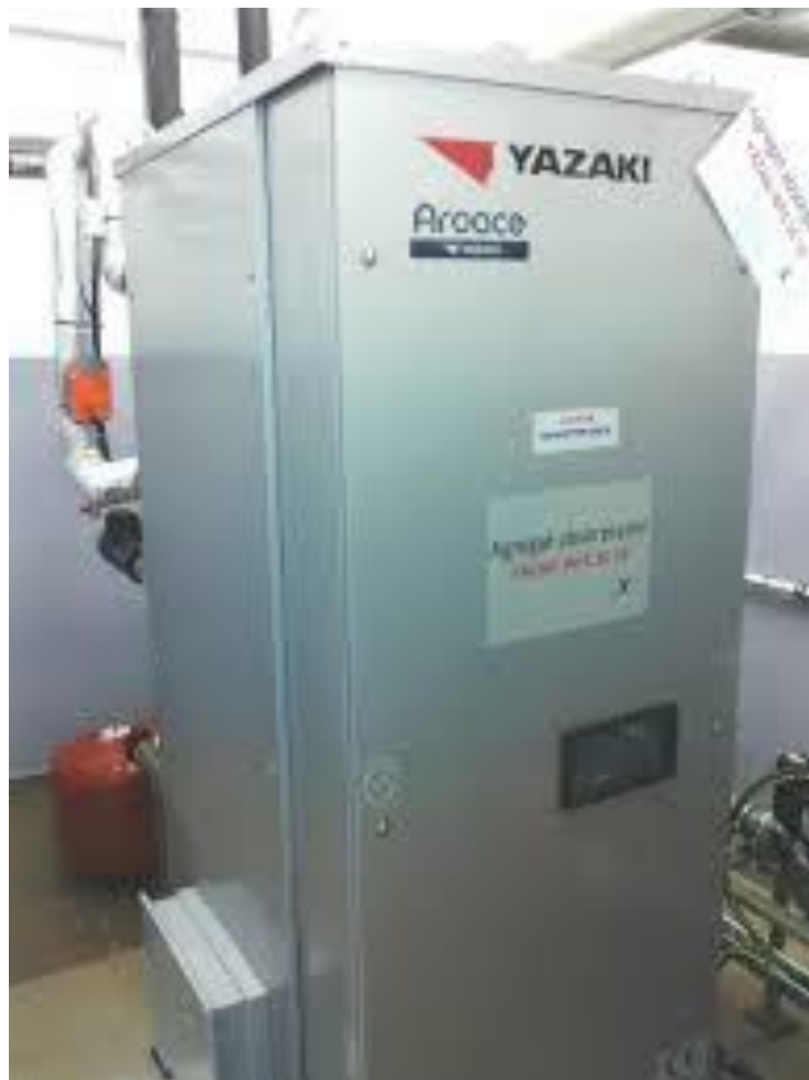
Figure 4 : Machine froide YAZAKI
