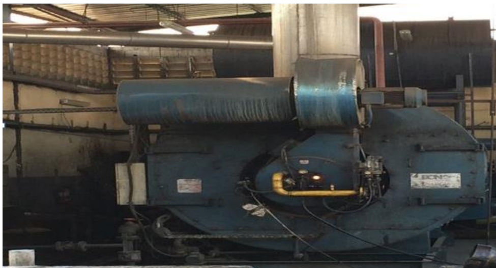
Figure 5: Chaudière BONO ENERGIE SG 1000
