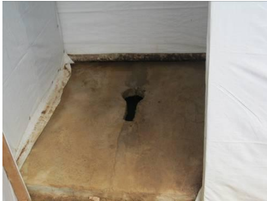
Picture 19: Before rehabilitation
