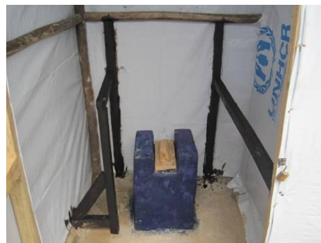
Picture 21: Rehabilitated latrine with seat and handrails
