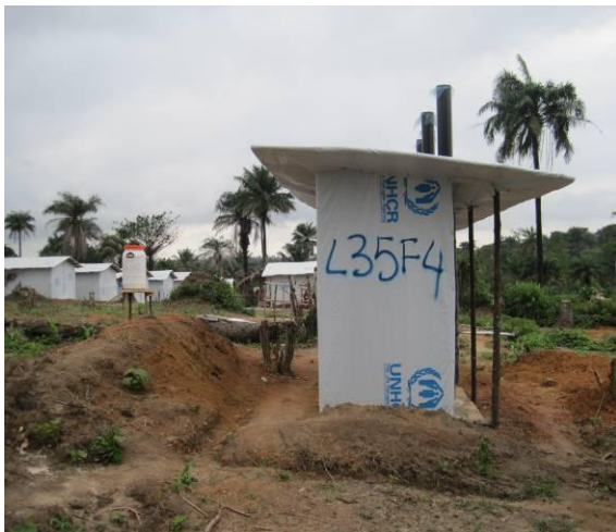
Picture 9: Drainage system around the latrine
