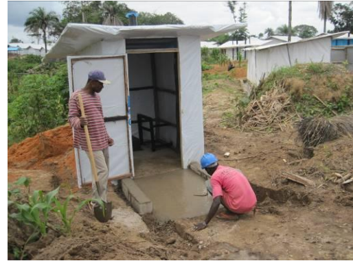
Picture 16: Ramp construction
