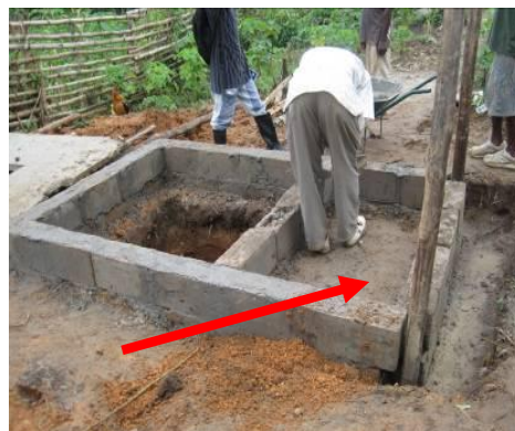
Picture 14: Column of bricks
