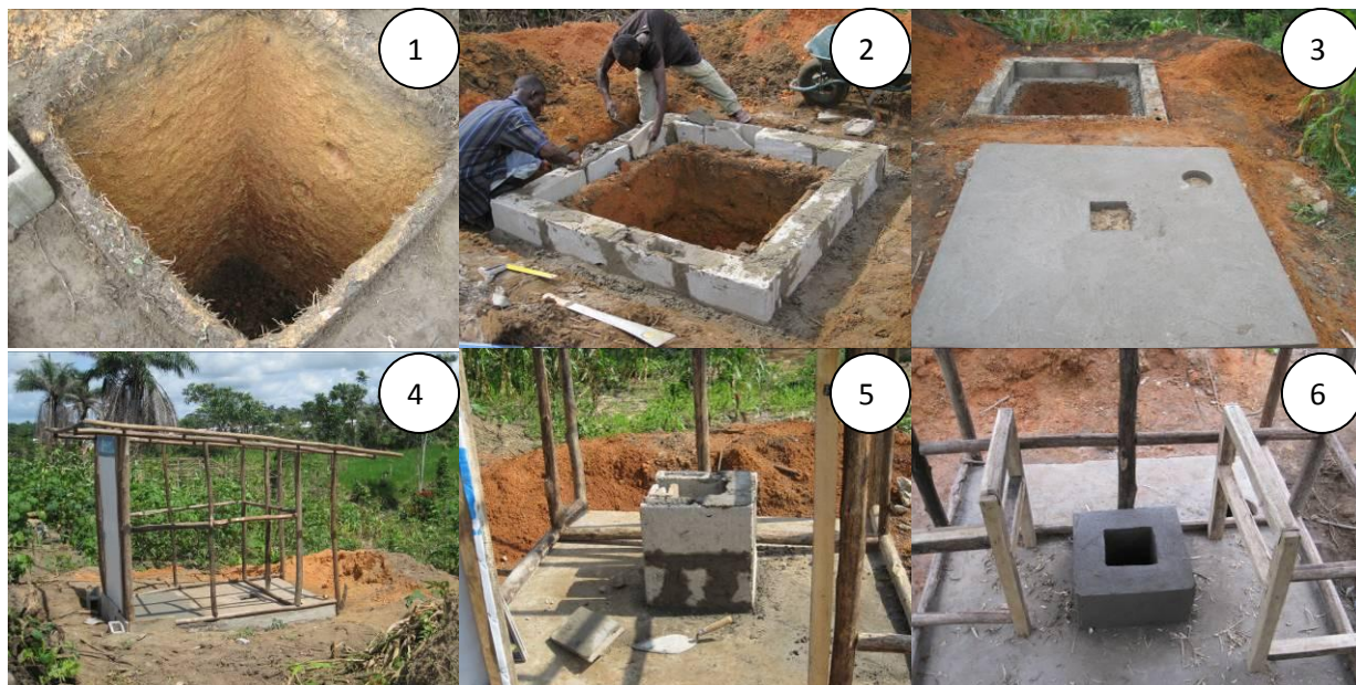
Picture 13: Structural work stages for vulnerable people's latrine construction
