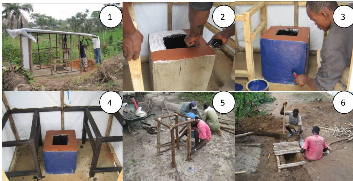
Picture 15: Finishing works for vulnerable people latrine
