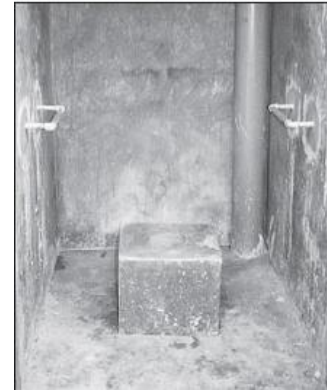
Picture 12: Source Hazel Jones & Bob Reed.(2005). Disabled people's latrine at Bubajjwe's school in Kampala, Uganda
