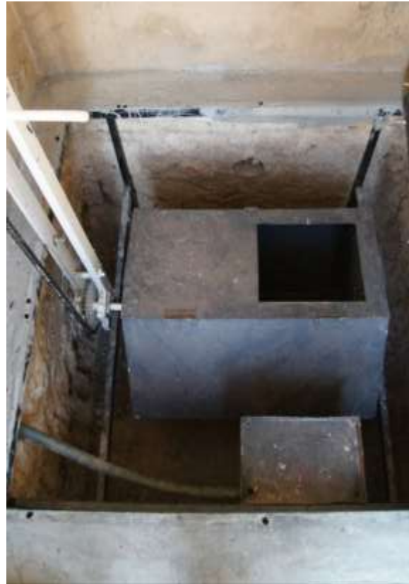
Figure 1. 5: Rural model composting toilet used in the study showing the inner view of the composting reactor (Source: R. Ito).
