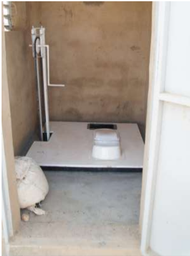
Figure 1. 5: Rural model composting toilet used in the study showing the inner view of the composting reactor (Source: R. Ito).
