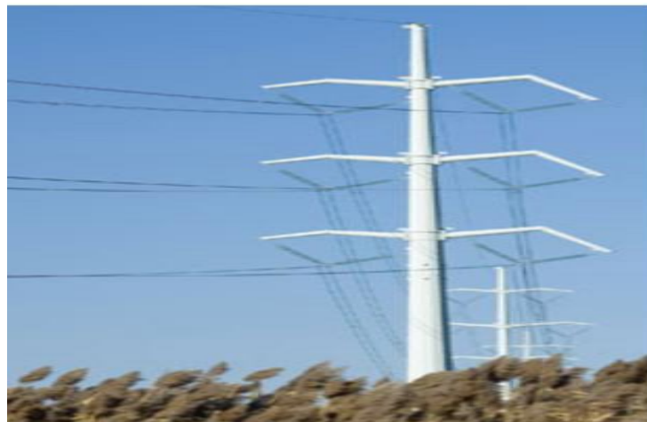
Figure 6 : Pylône monomode
