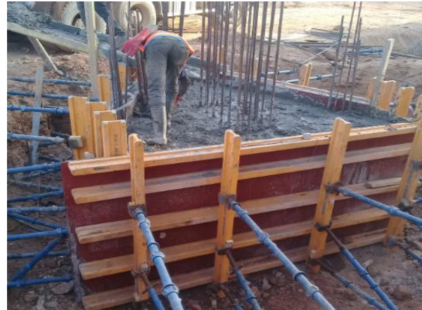
Figure 23: Coffrage de la semelle
