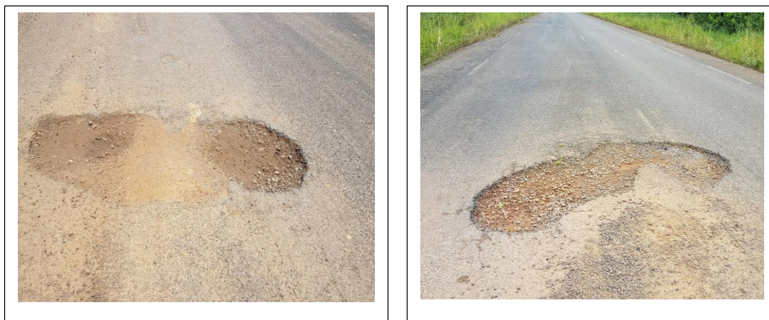
Figure 6: images illustratives des nids de poule
