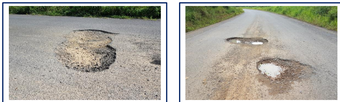
Figure 7 : illustration nids de poule
