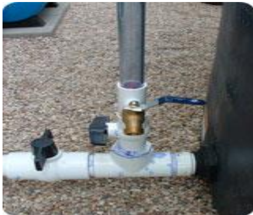
Image 3: first flush water diverter
