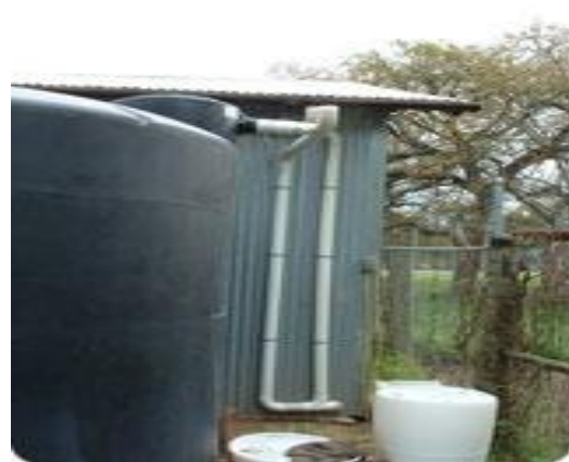
Image 4: clear or transparent water level indicator pipe
