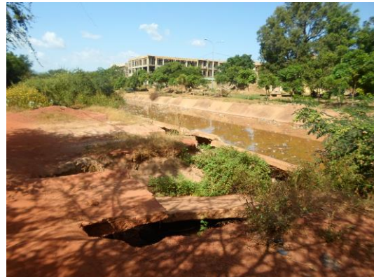
(B) Unrehabilitated channel sides
