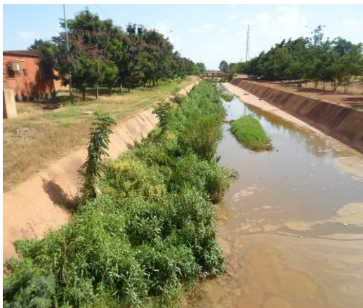
(C) Plants growing into the channel
