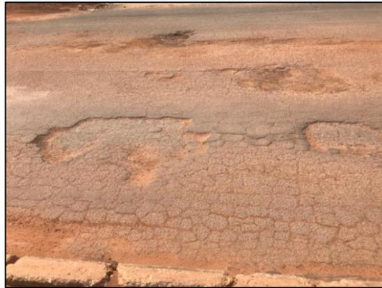
*Figure 6: Photo illustrative des fissurations maillées + arrachement*
