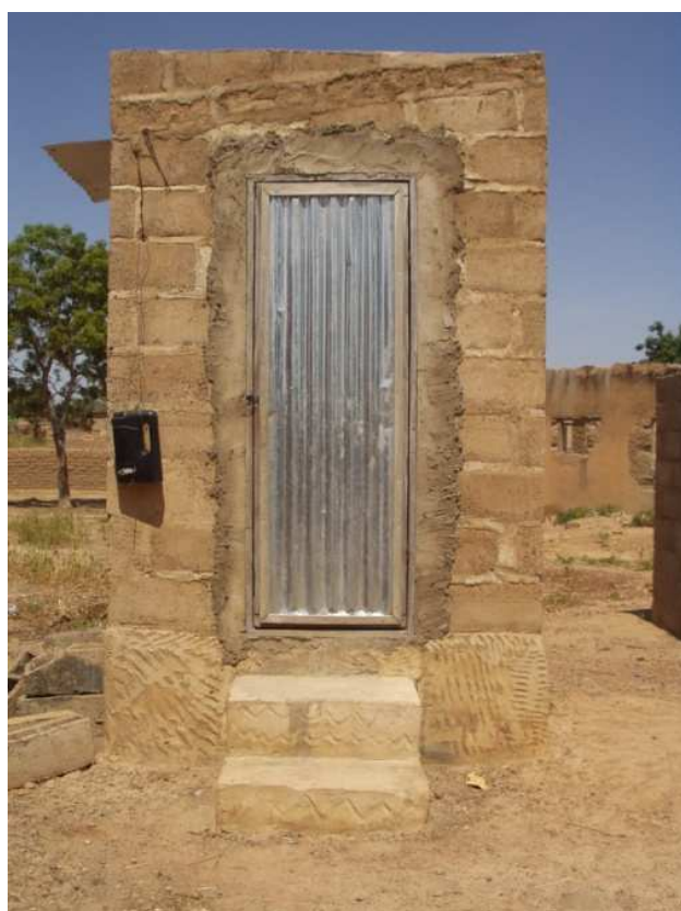
Figure 3-a: Latrine type Tecpan (vue avant)
