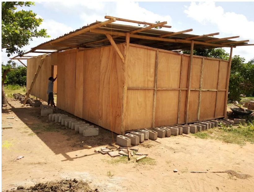
Figure 6: Photo baraque Chantier de Zatta 2
