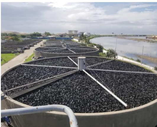
Figure 3-G: The Trickling Filters
