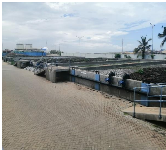
Figure 3-I: The Sludge Drying Beds
