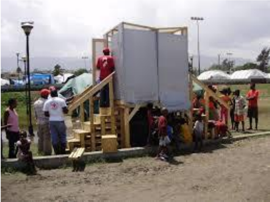
Fig 10 Elevated Pit Latrine Installation in an IDP Camp (Internet Sourced)
