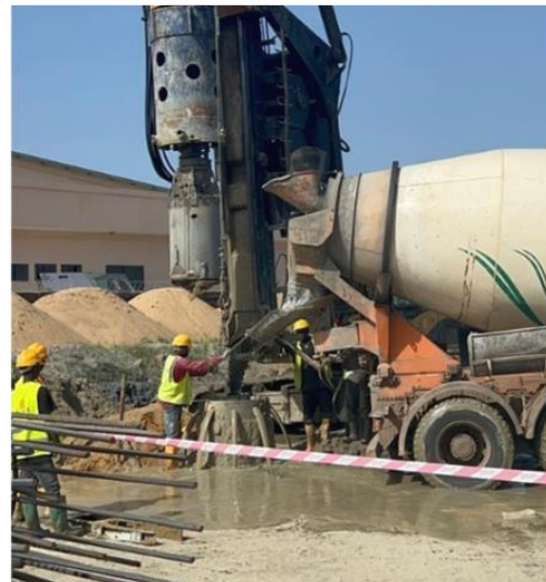
Figure 8: Coulage du pieu
