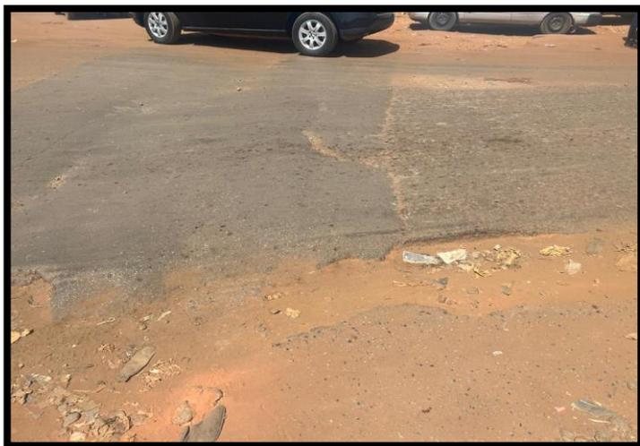
Figure 12: Fissuration Transversale PK0+950
