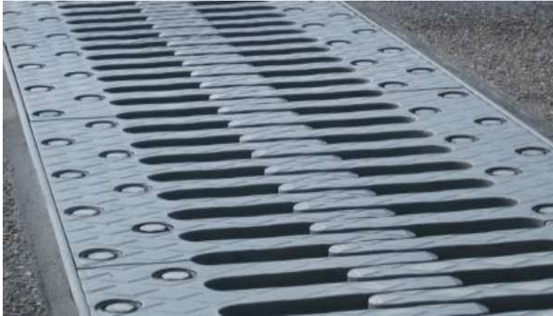
Figure 6: Joint de chaussée
