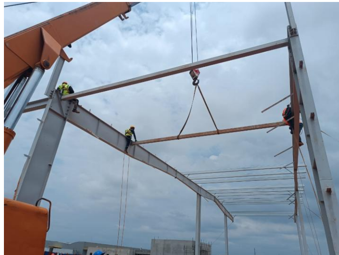
Figure 6: Installation des pannes
