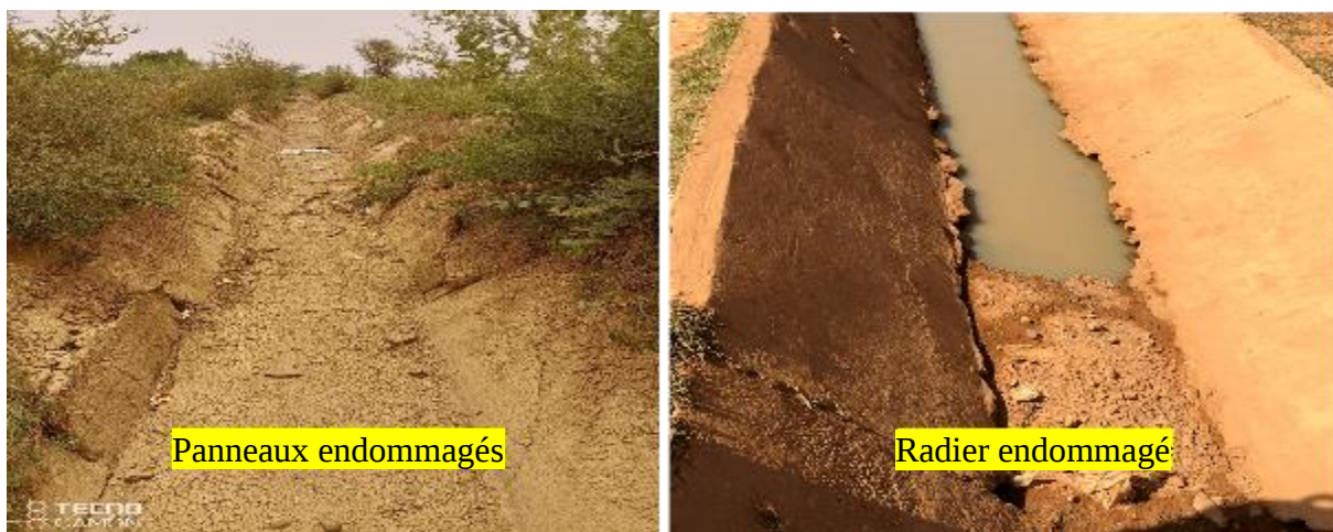
Figure 7 : Canal principal (CP)
