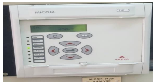
Figure 23: Relais Micom AREA
