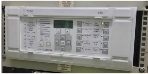
Figure 24: Relais de protection Micom ALSTOM
