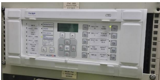
Figure 22: Relais de protection Micom ALSTOM
