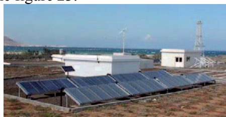
Figure 23. View of the solar collectors field coupled to the H/D desalination system.
