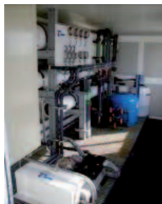
Figure 28. SWRO desalination plant. Container housing SWRO unit.
