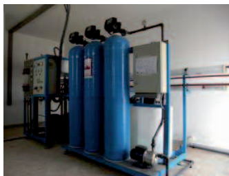
Figure 21. RO unit installed in Morocco.
